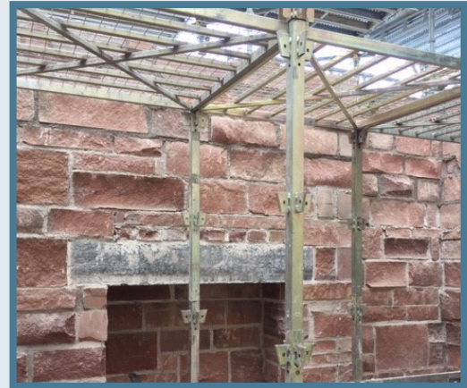
Fountainbridge Tenement Reinstatement, Edinburgh, £1.45 million. This building consists of 15 flats and three retail units at ground level. Our stonework repairs are progressing well under a temporary roof.
