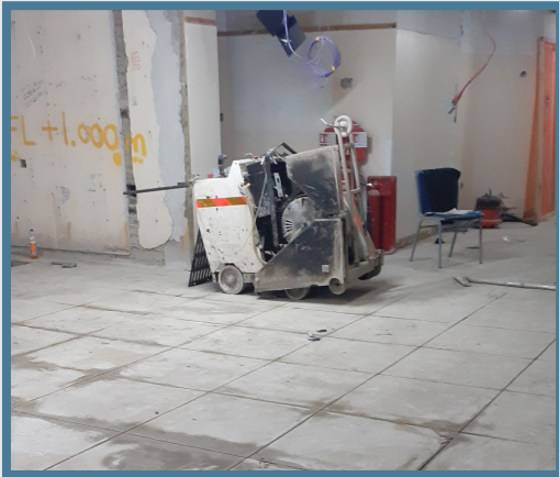
Thrombectomy Suite at Queen Elizabeth University Hospital, Glasgow, £2.2 million. We are replacing two redundant operating theatres within the existing Institute of Neurological Sciences with the new thrombectomy suite. Our team is cutting out the existing concrete floor to accommodate plant and equipment for the new procedures room.
