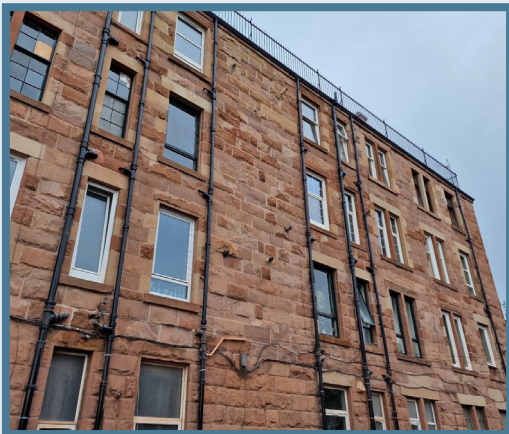
Camphill Gate External Refurbishment, Pollokshaws Road, Glasgow, £1.4 million. Our scaffolding has now been removed on the tenement's rear elevation showing completed stone repairs, and wrought iron balustrading to the flat roof to this B listed building. The front elevation will be revealed soon.
