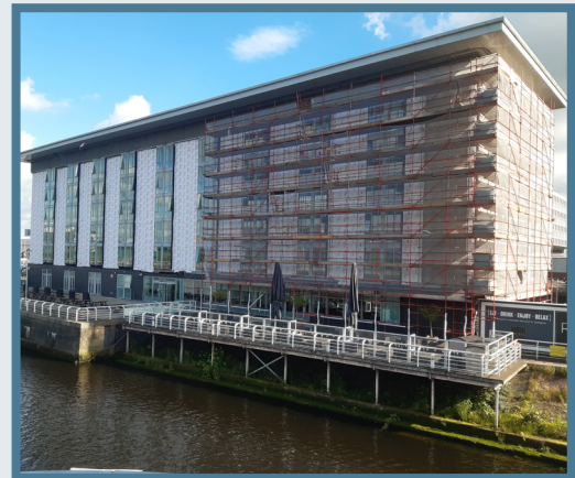
Hilton Garden Inn External Refurbishment Project, Glasgow, £2.2 million - scaffolding is being erected ready for work to begin.
